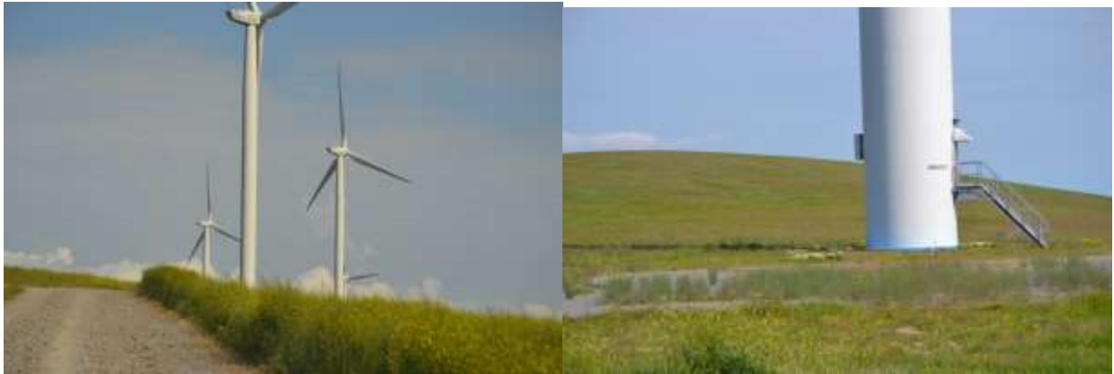
Fig. 7-8: drum acces si platforma turbina
